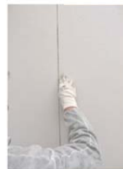
Joint de dilatation 3 mm
